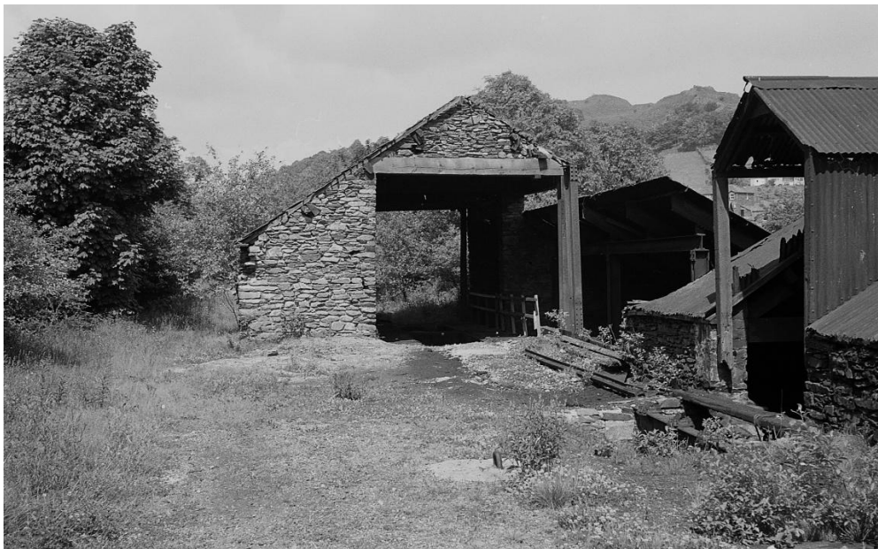
Peter Holmes img067. Taken from further along the lifted tracks. It shows the line passing over the chute into one of the storehouses (to the right), before entering the covered area for unloading iron ore.
